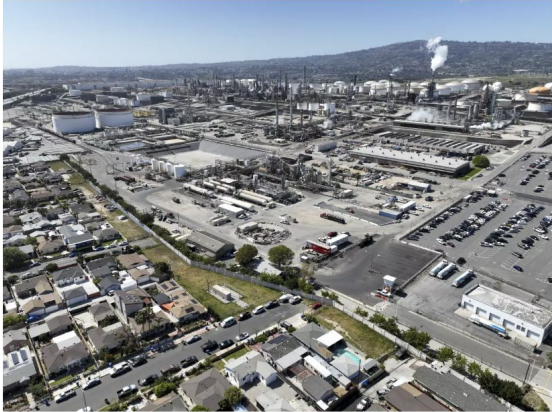
The Phillips 66 refinery in Wilmington in 2022. (Allen J. Schaben / Los Angeles Times)
