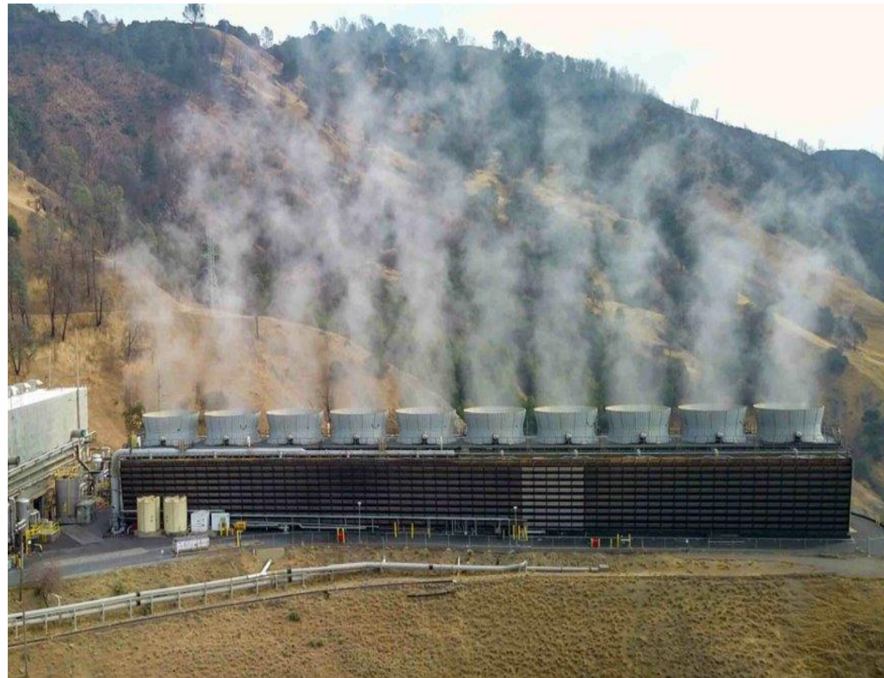
Geysers Geothermal Power Plant 955 MW
