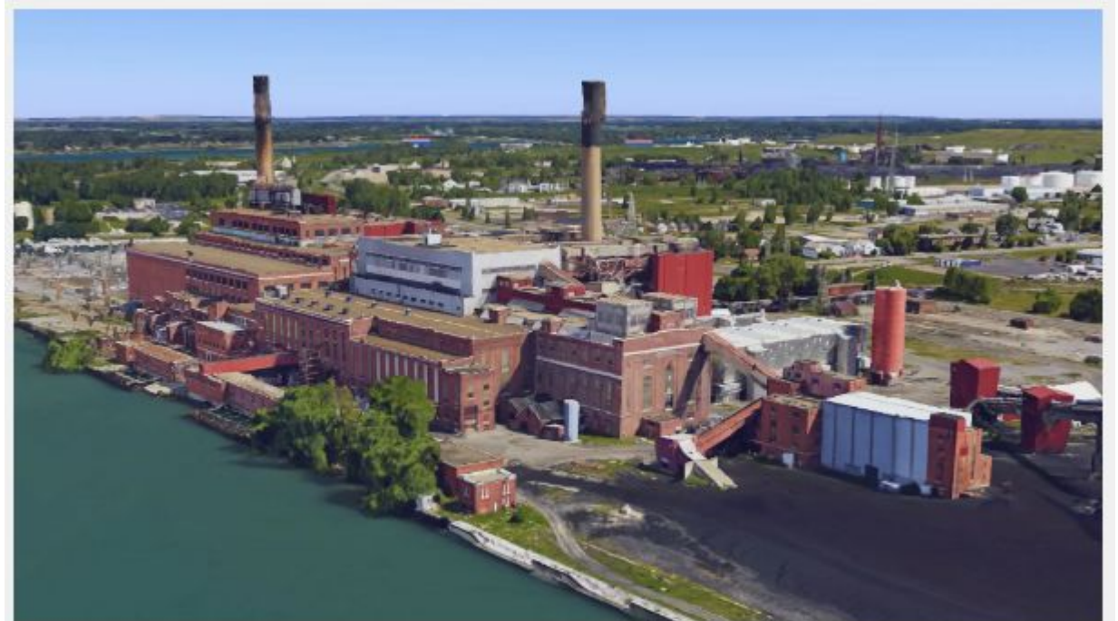
The retired Huntley Generating Station on the banks of the Niagara River. Google Earth
