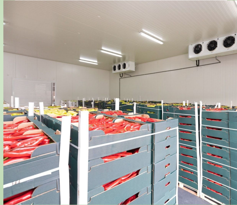
Porterville Cold Storage Facility
