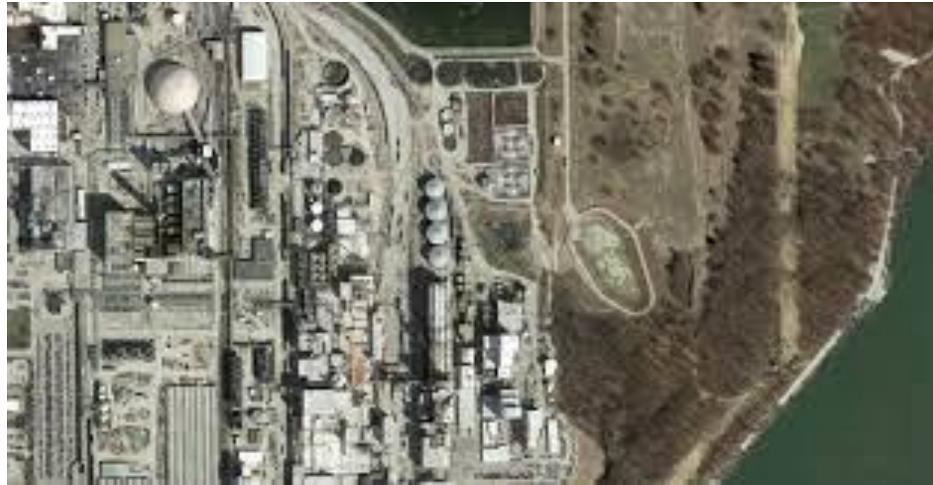
Archer Daniels Midland Illinois BECCS facility
