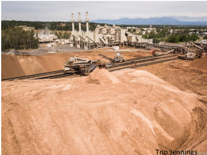
Chip storage piles emitting methane
