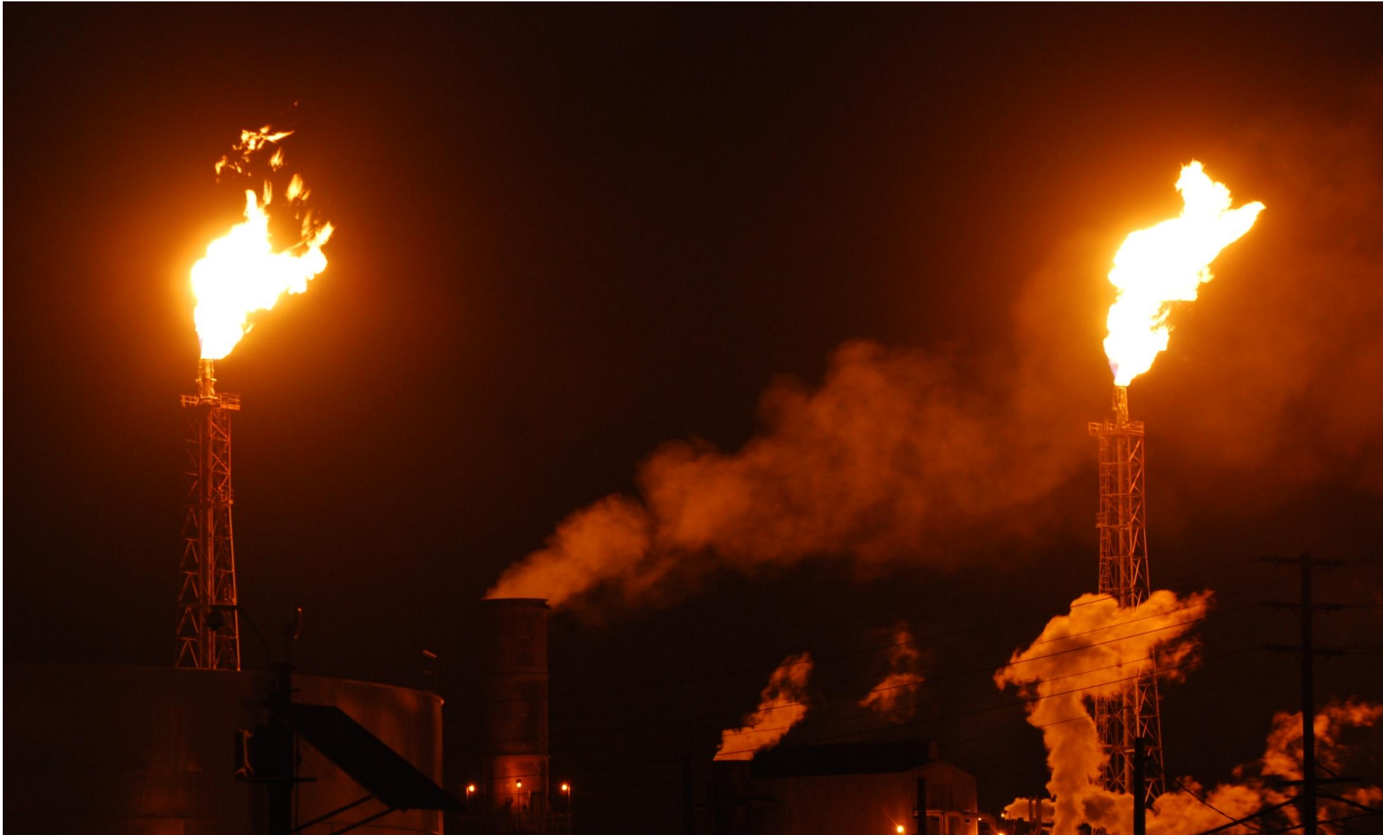
3-9-2010 Tesoro Wilm. Power Outage caused Flaring, billowing smoke, neighbors reported explosions, AQMD told us they had no equipment for air samples that night
