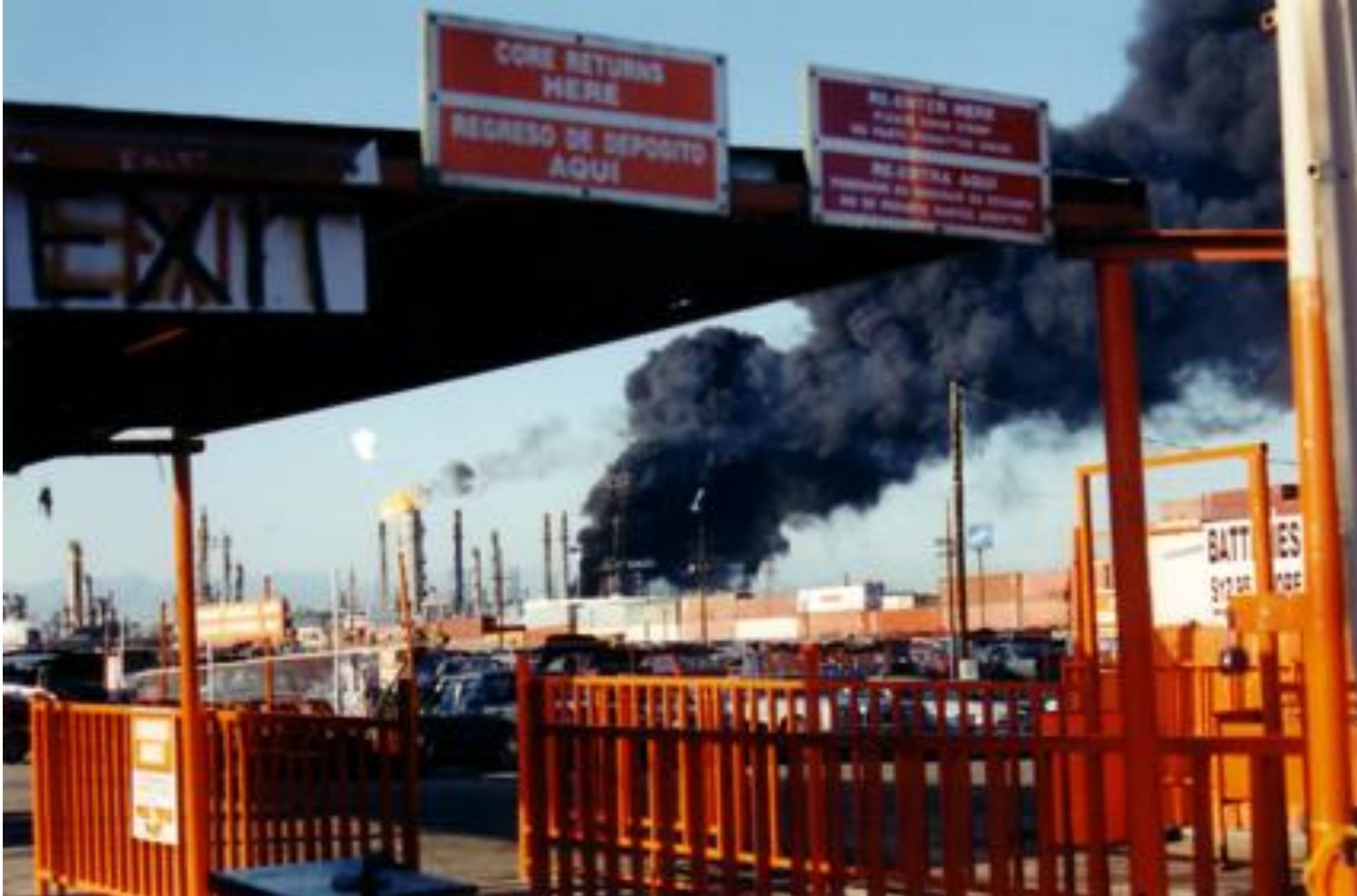
April 23, 2001- Tosco Refinery explosion & fire, Carson – another coker fire
