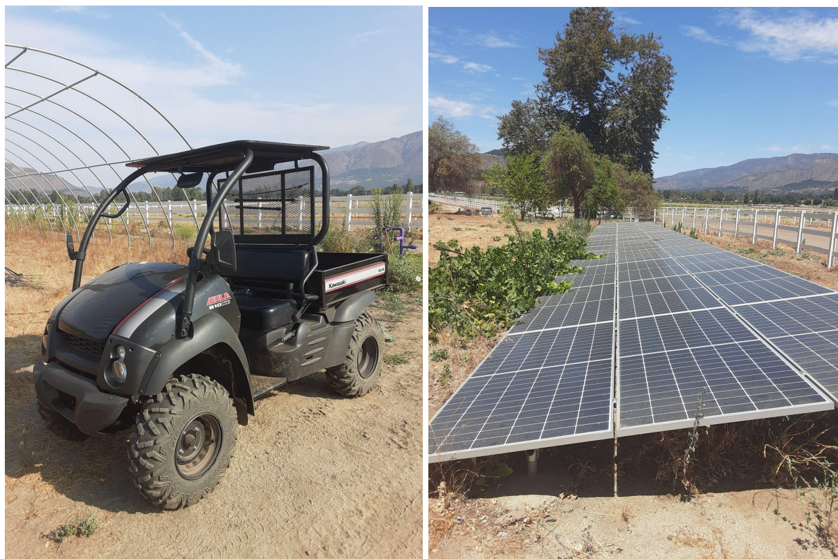
Figure 16 & 17, Kawasaki Mule & Solar panels array
