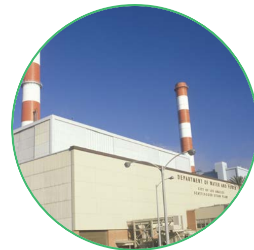
Clean, Dispatchable Power Generation
