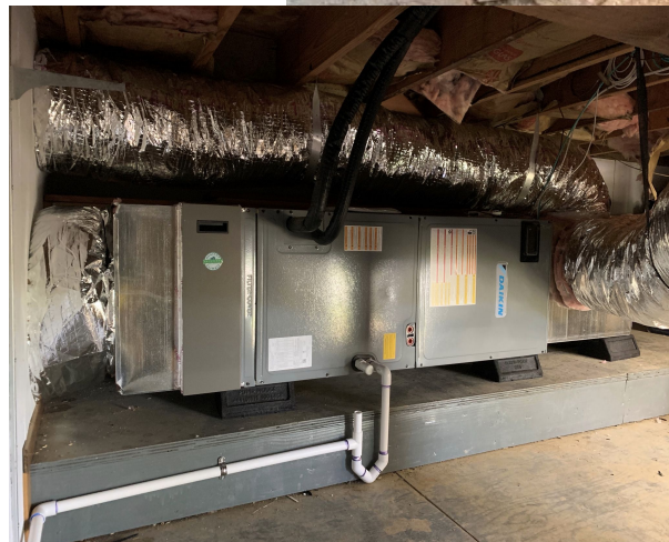
Split system heat pump HVAC system: outdoor & indoor units
