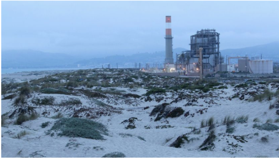
The Mandalay generating station at Mandalay Beach in Oxnard. (Myung J. Chun / Los Angeles Times)
